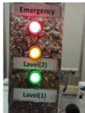
Figure 28: level indicator lamps in the emergency state.
